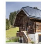
2020.05.22 Single Family House Switzerland
