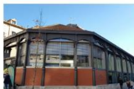
2019.07.03 Mercado del Val, Valladolid (Spain) Spain
