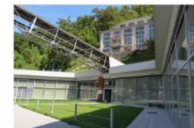
2019.10.08 Idrija mercury smelting plant Slovenia
